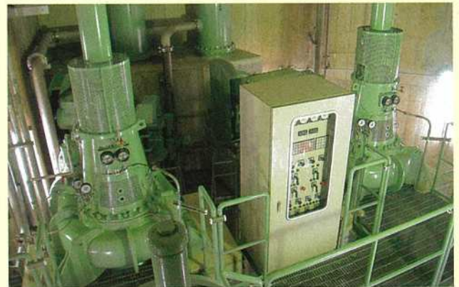
Main discharge pump of Zenpukuji River intake facility
