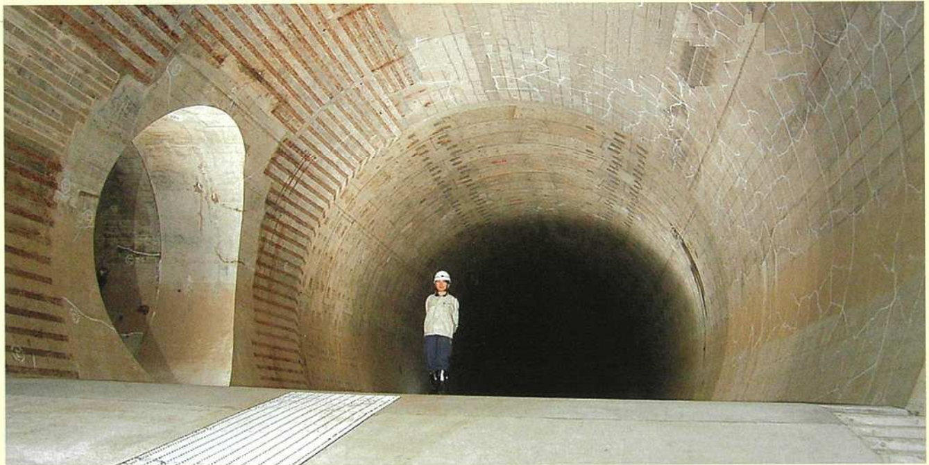
Zenpukuji River intake facility connecting duct joint points of the Stage 1 tunnel
